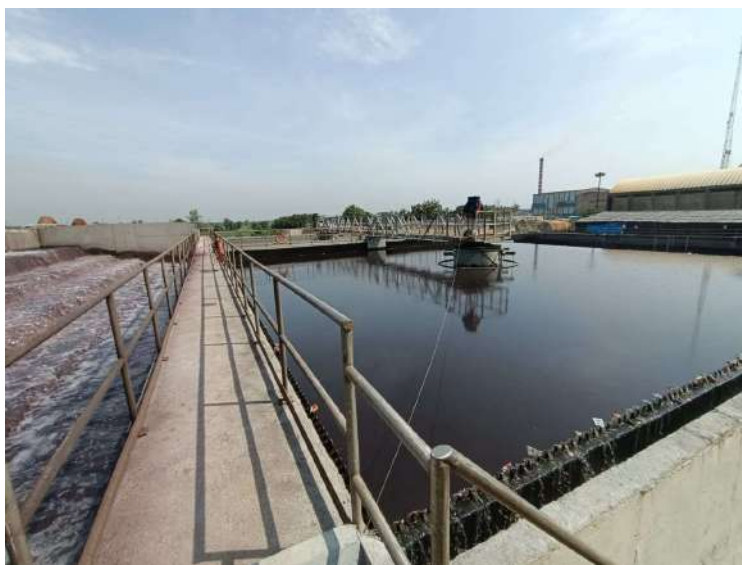
Figure 3.4 New Pre-Sedimentation Tank
